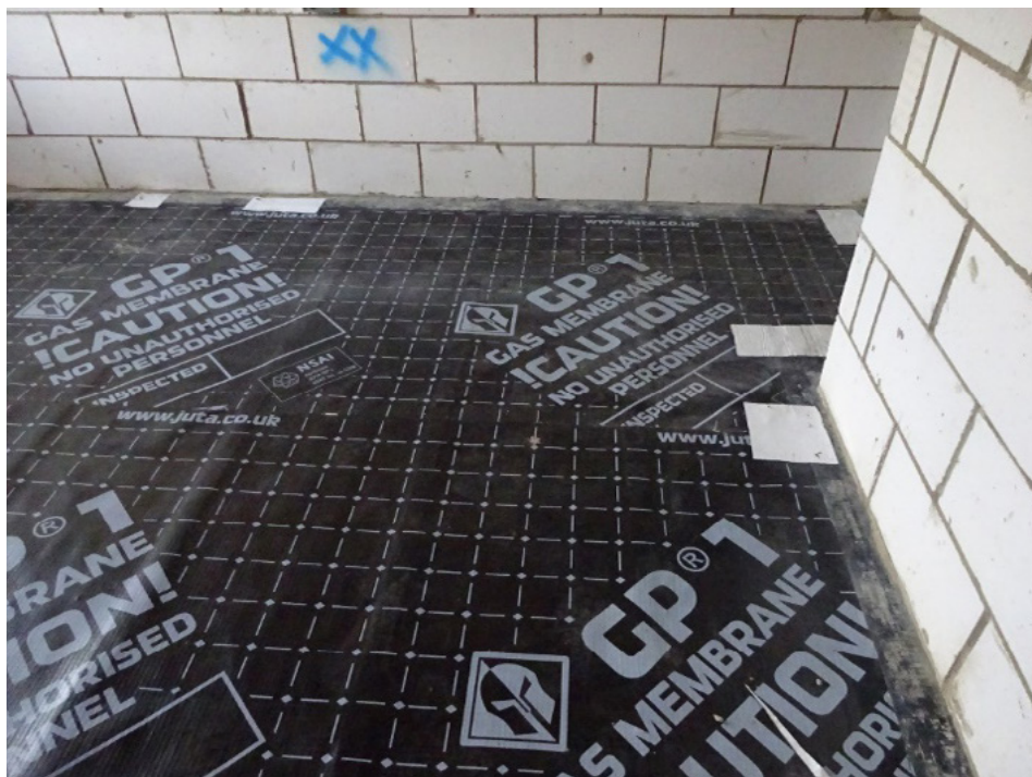
Figure C6 Perimeter cavity membrane with main infill membrane - with infill membrane completed
